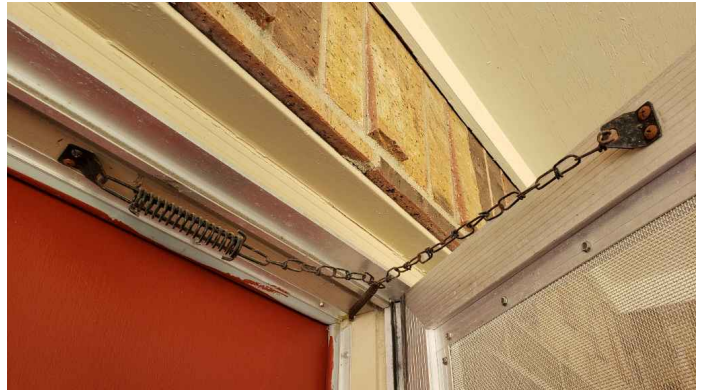
Door safety swing catch and chain. Many units are missing or have broken clasps.
