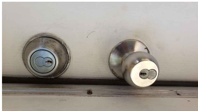
Ext Door (Outside Profile) with door knob, keyed deadbolt and 1/2 bore for interior privacy deadbolt.
