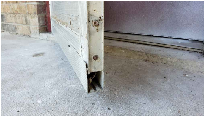
Bottom door hallow chamber that will need to be cleaned/washed out.
