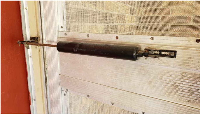
Door closure. Many units are need of replacement as do not function properly.
