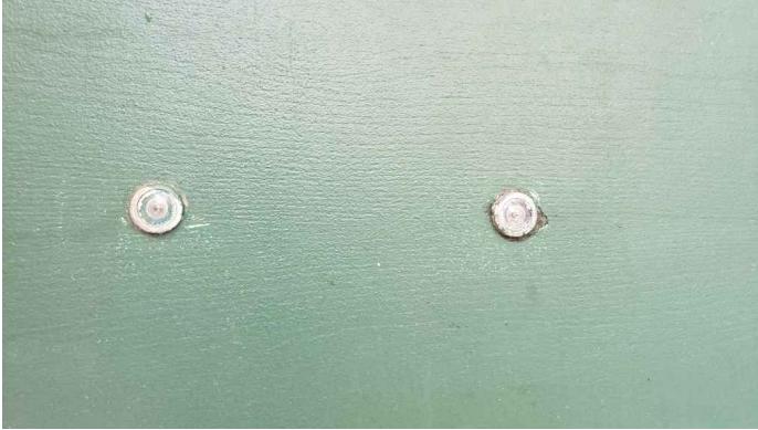
ADA Units require 2 peepholes on Exterior Doors.
