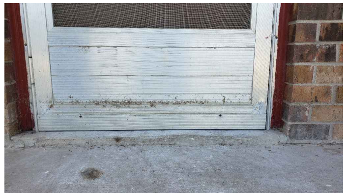
Avg Flood Line on Screen Doors
