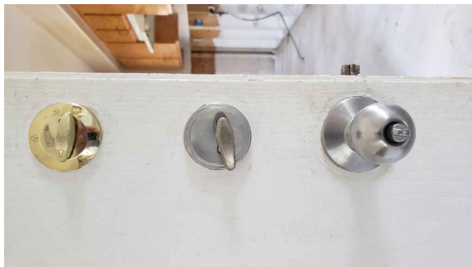
Ext Door (Interior Profile) with door knob, keyed deadbolt and 1/2 bore for inside privacy deadbolt (pictured on top)
