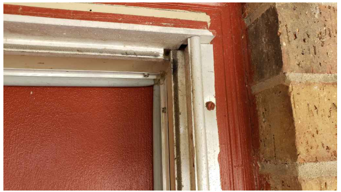
Frame and Mounting screwed into door jamb.
